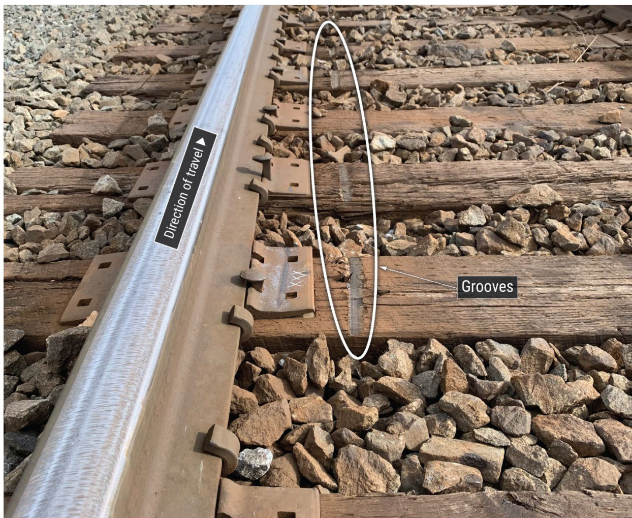
Figure 12. Wheel flange marks on cross-ties east of MP 49.5.
