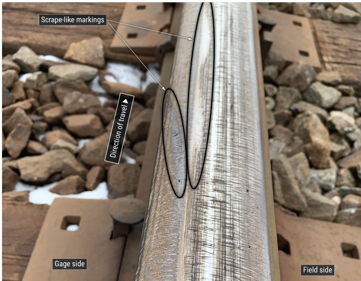
Figure 11. South running rail at MP 49.5.
